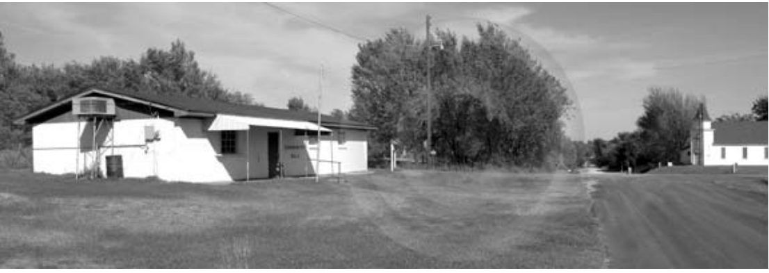
The community center, left, and the First United Methodist Church, right, are the only two vintage structures still in use in Bridgeport, Oklahoma.
